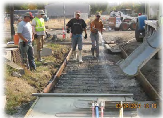
Sidewalk Construction in Roundup
