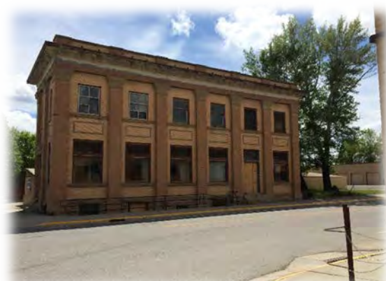
Old Bank Building
