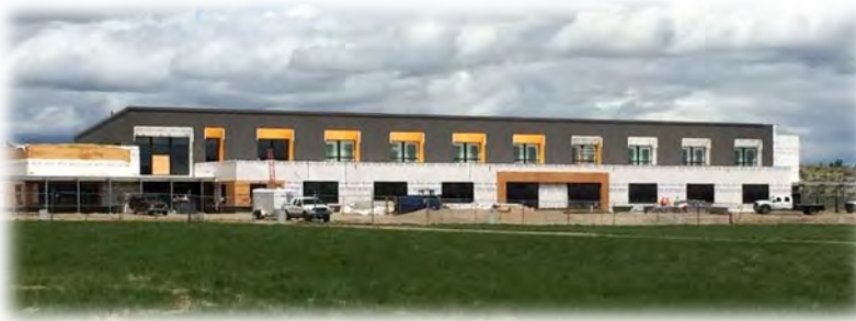
New Elementary School Under Construction
