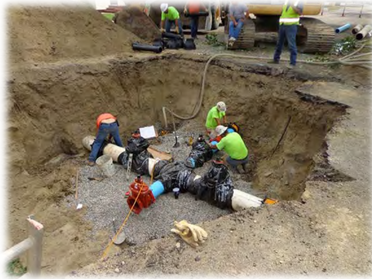
Installing New Waterlines in Roundup
