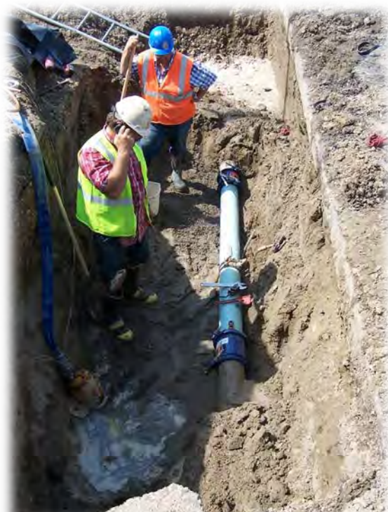
Water Line Repair in Roundup
