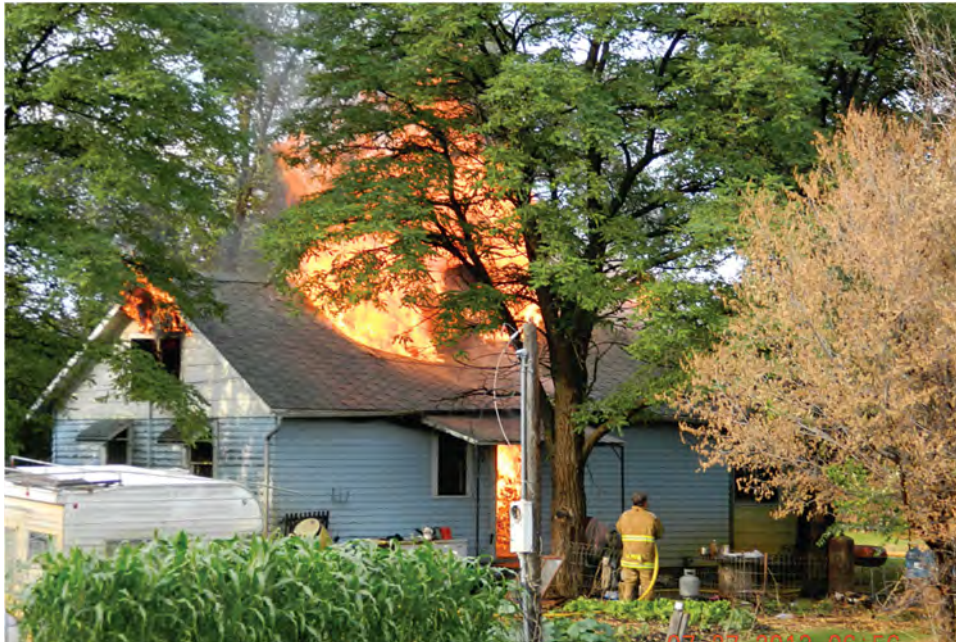
Figure 2.5: Home Destroyed by Fire July 2013
