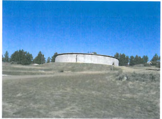
Storage facility (ST001)
