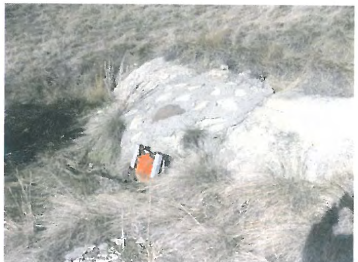
Storage tank drain and overflow pipe (ST001)
