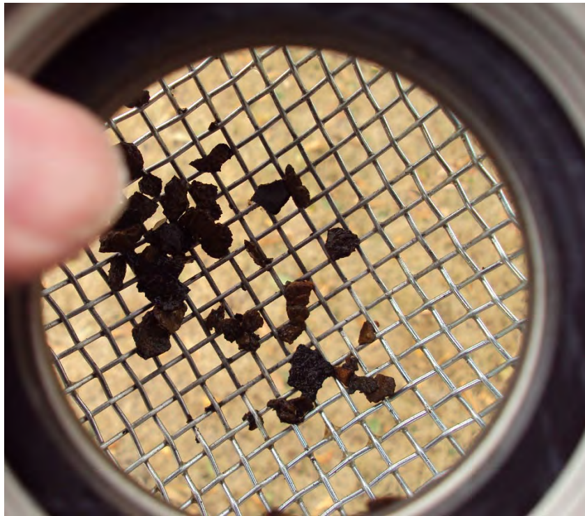
Figure 4.2: Rust Particles in Fire Department Screen
