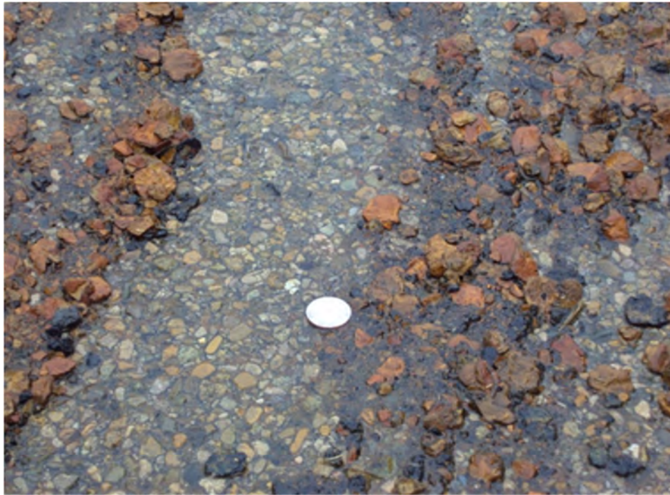
Figure 3.7: Material Present in Flow from Cast Iron Water Mains
