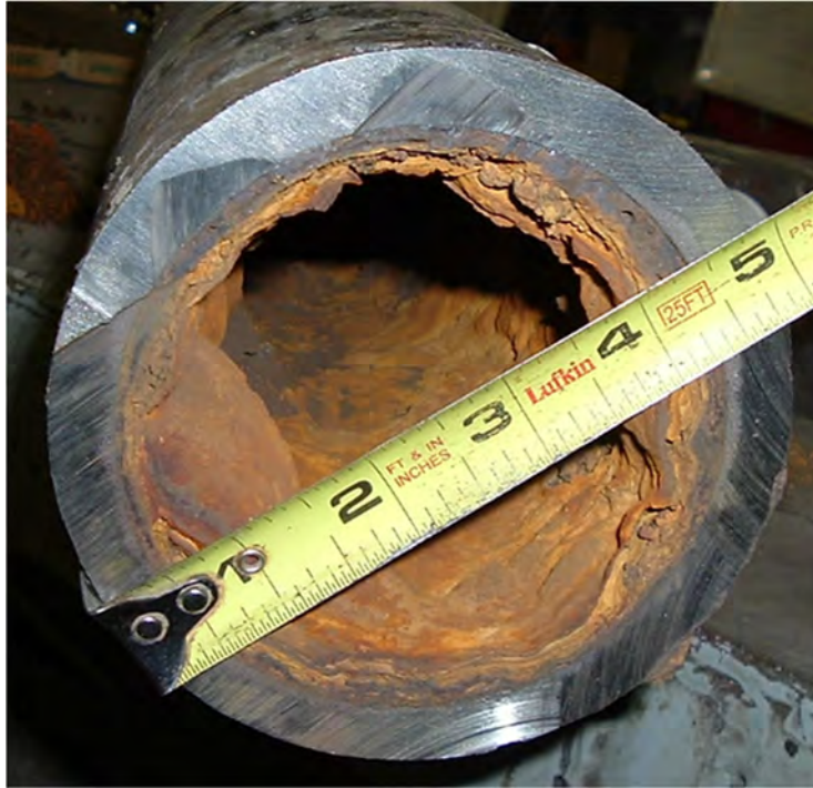
Figure 4.1: Typical 4-Inch Cast Iron Main Removed Due to Break
