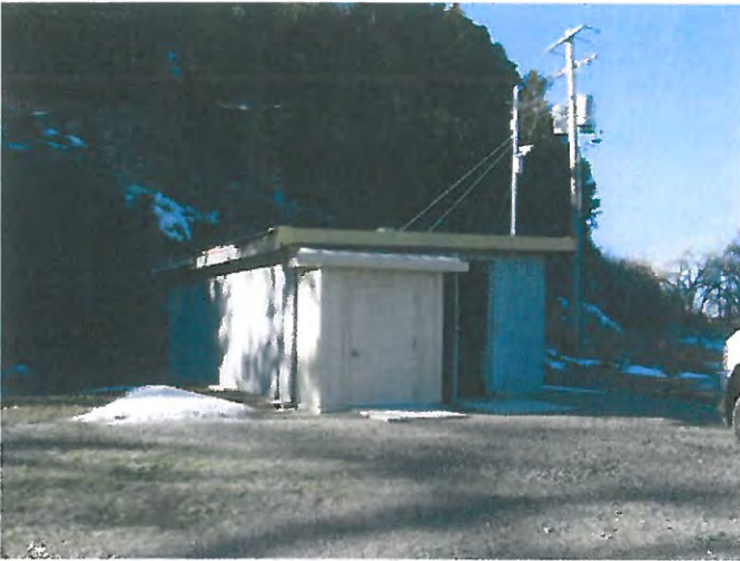
Pump house containing well pumps, telemetry pump controls, and treatment plant. The common header is buried on west side of building.
