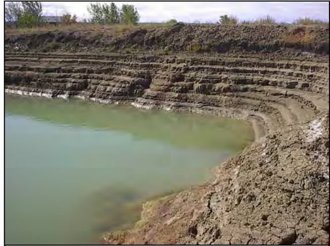
Figure 3.5: Emergency Storage Pond
