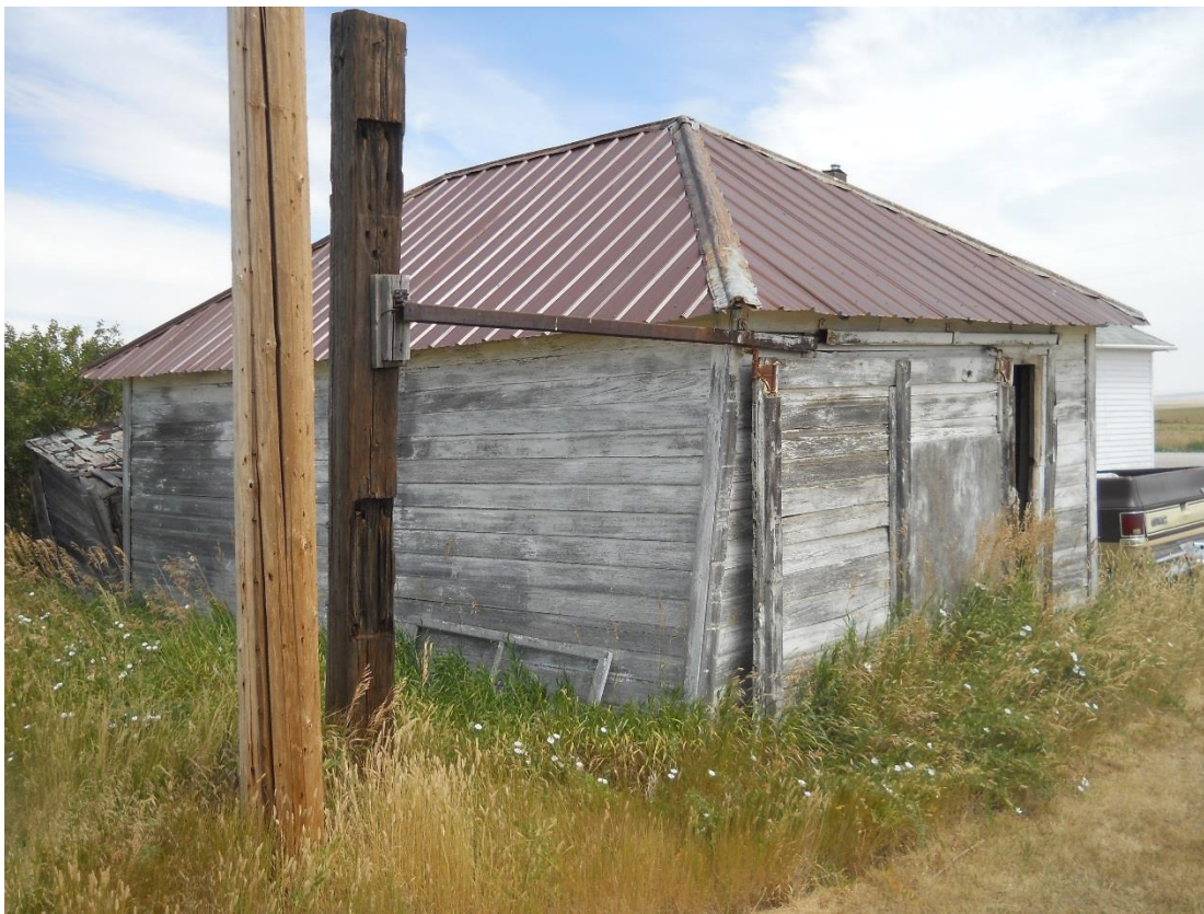
Feature 3, Garage, View to the Northeast.
