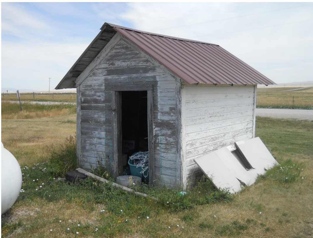
Feature 2, Shed, View to the Northeast.
