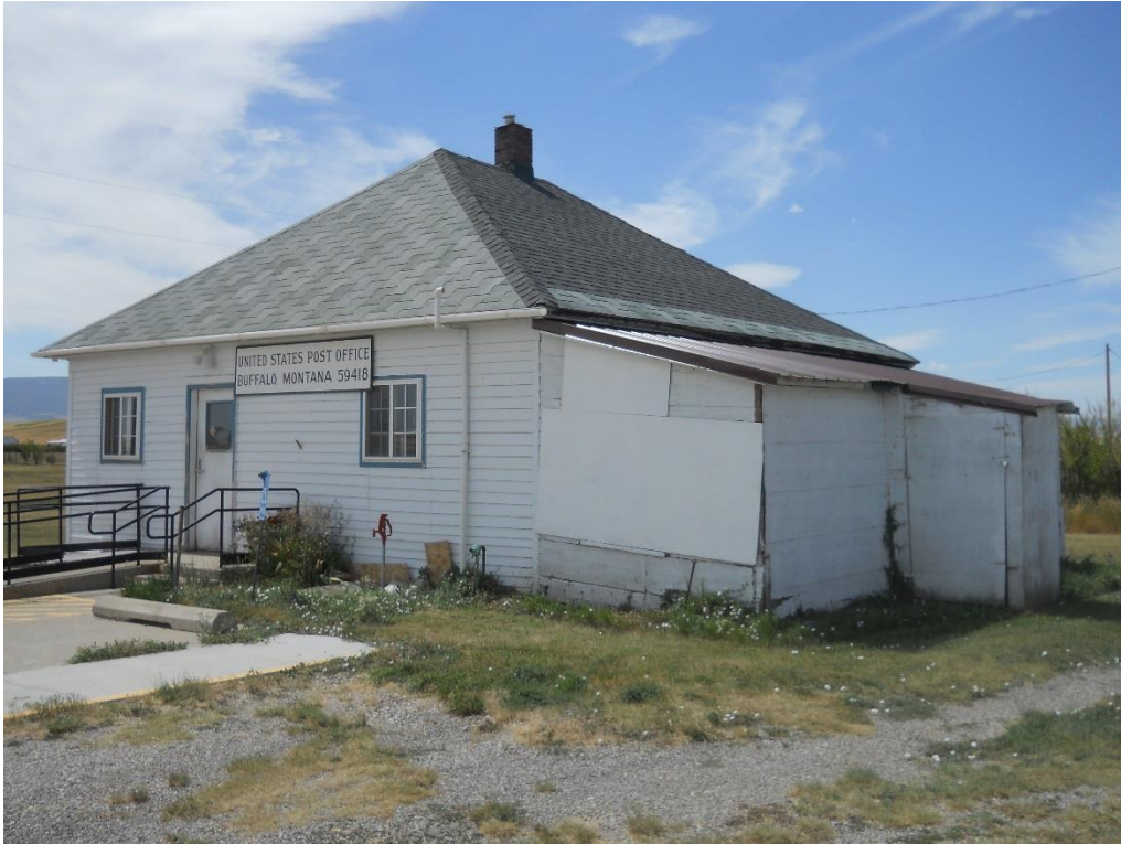
Feature 1, Residence/Post Office, View to the Southwest.
